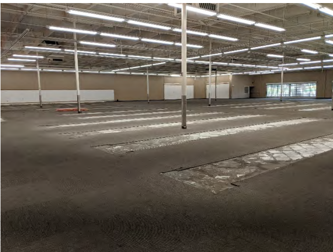
Photo 11: Interior of former Office Max store.
