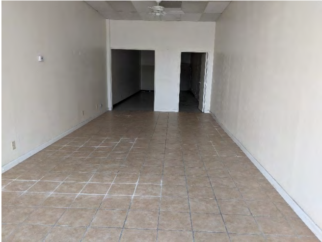
Photo 13: Interior front portion of former dry cleaner tenant space at 5580 Unit C.
