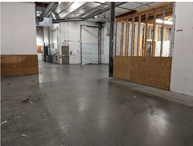
Photo 9: Rear interior area of former Office Max store.
