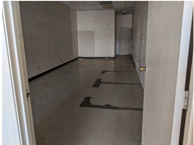
Photo 14: Interior rear portion of former dry cleaner tenant space at 5580 Unit C.
