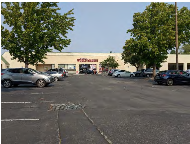
Photo 3: Parking lot and front exterior of Cost Plus World Market building.
