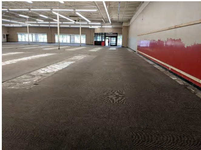
Photo 12: Interior of former Office Max store.
