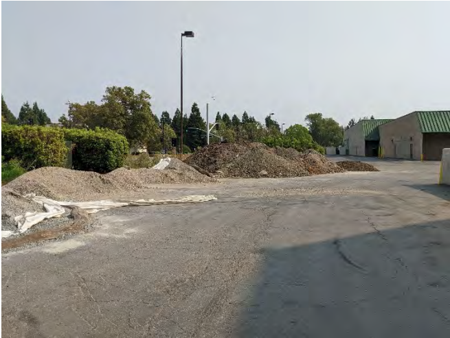
Photo 7: Soil piles and miscellaneous debris associated with City improvement work; east portion of property.
